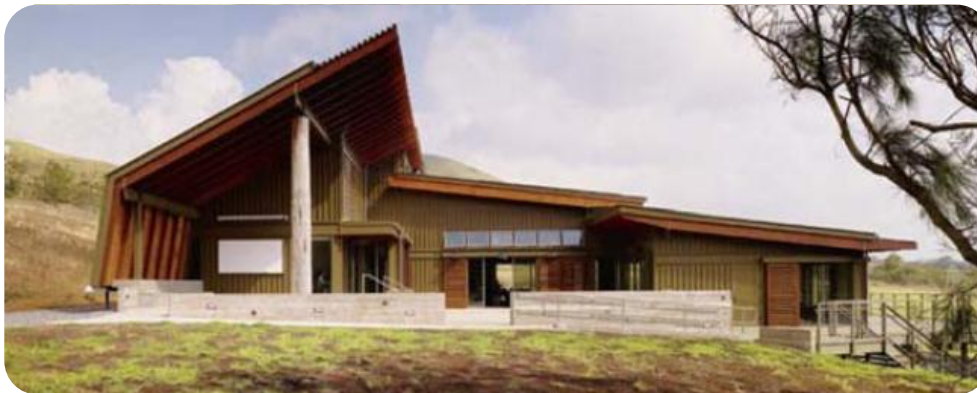
The Energy Lab , Kamuela Hawaii
